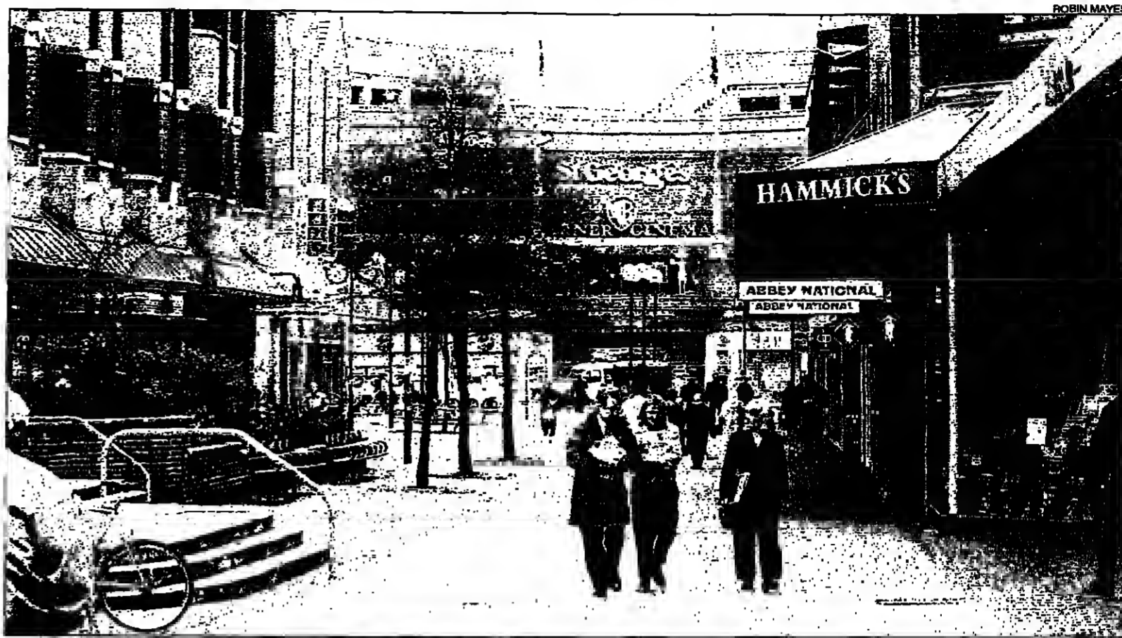
Harrow's £40 million St George's shopping and leisure centre that opens tomorrow: it features a cinema and family entertainment complex
